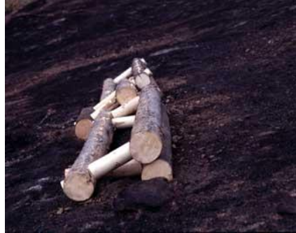
Figure 1. Conceptual smallwood erosion control structure is comprised of three poles connected by wood spars with round mortise and tenon joints.
