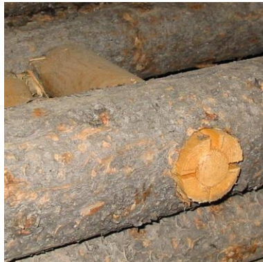
Figure 2. Round mortise and tenon joint uses a round cedar wedge to lock the spar to a pole.
