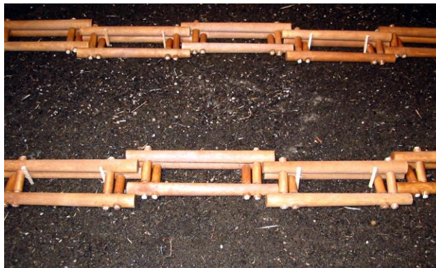
Figure 10. Staking of FlowCheck™ structures can be achieved by driving two stakes behind the upslope face of the lower set of structures in each run. Note that the upslope unit is held from movement by the overlap with lower units on either end.
