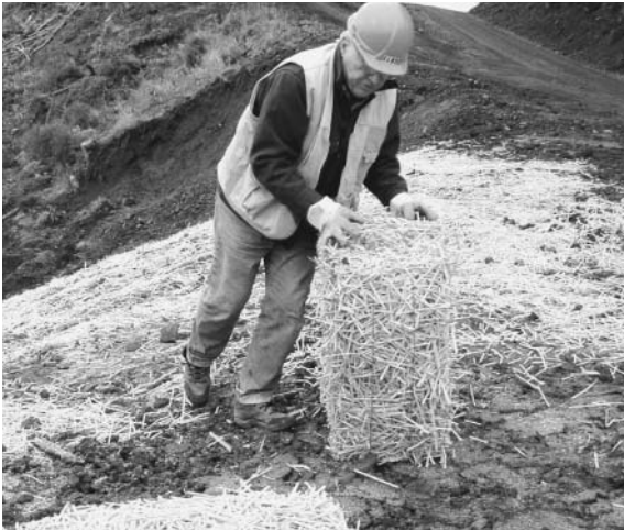
Wood-strand mulch is “weight-easy,” baled for handling on small projects like Weyerhaeuser’s forest road maintenance. (Photos by M. Brooks)
