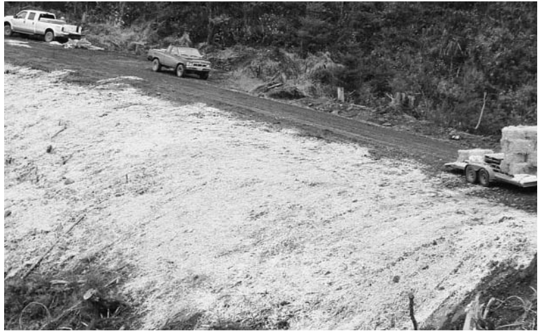
Wood-strand mulch is “weight-easy,” baled for handling on small projects like Weyerhaeuser’s forest road maintenance. (Photos by M. Brooks)
